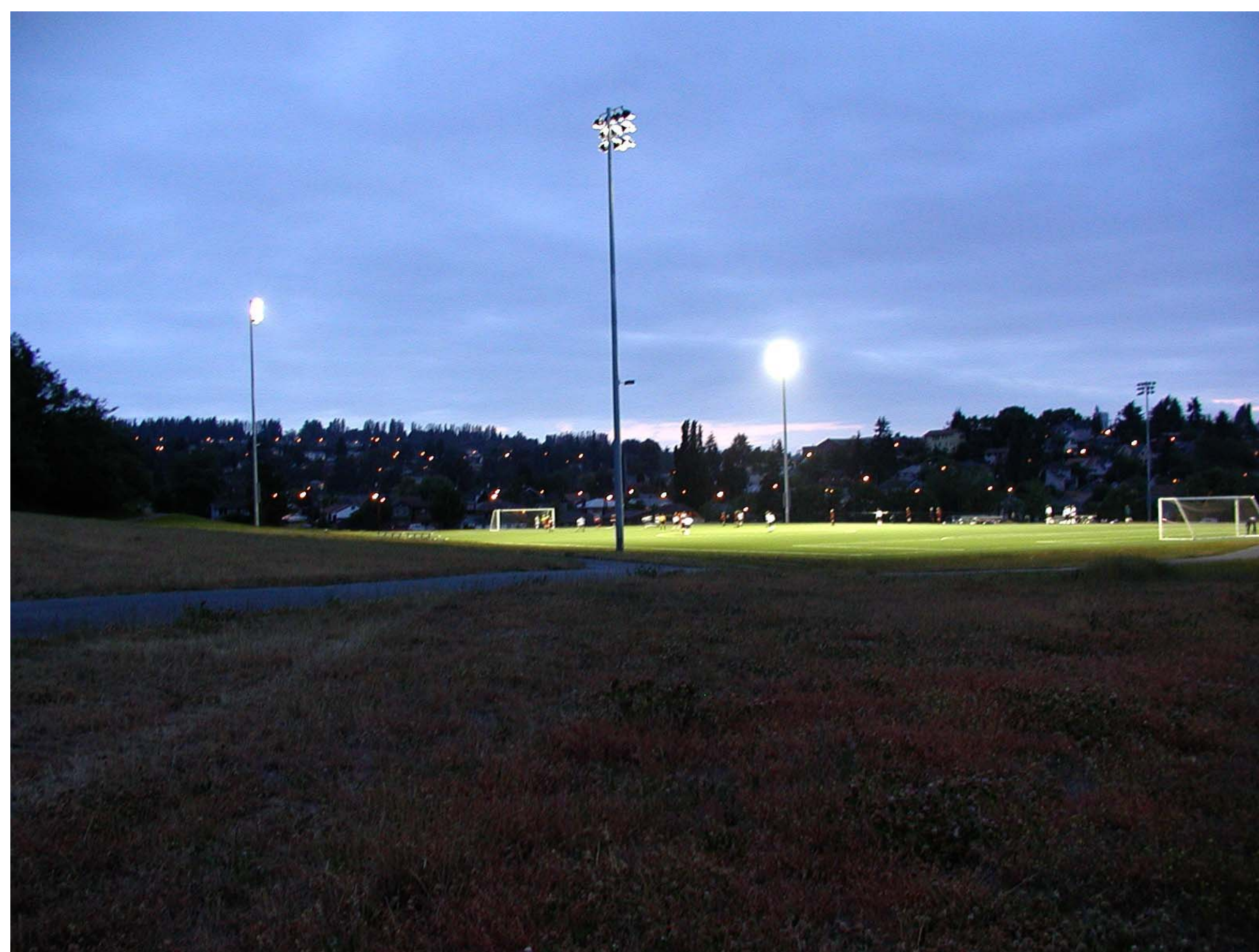
Urban soccer field with 4th generation spill and glare control fixtures illuminated to 300 lux. Photo taken approximately 50 metres from the edge of the field.
