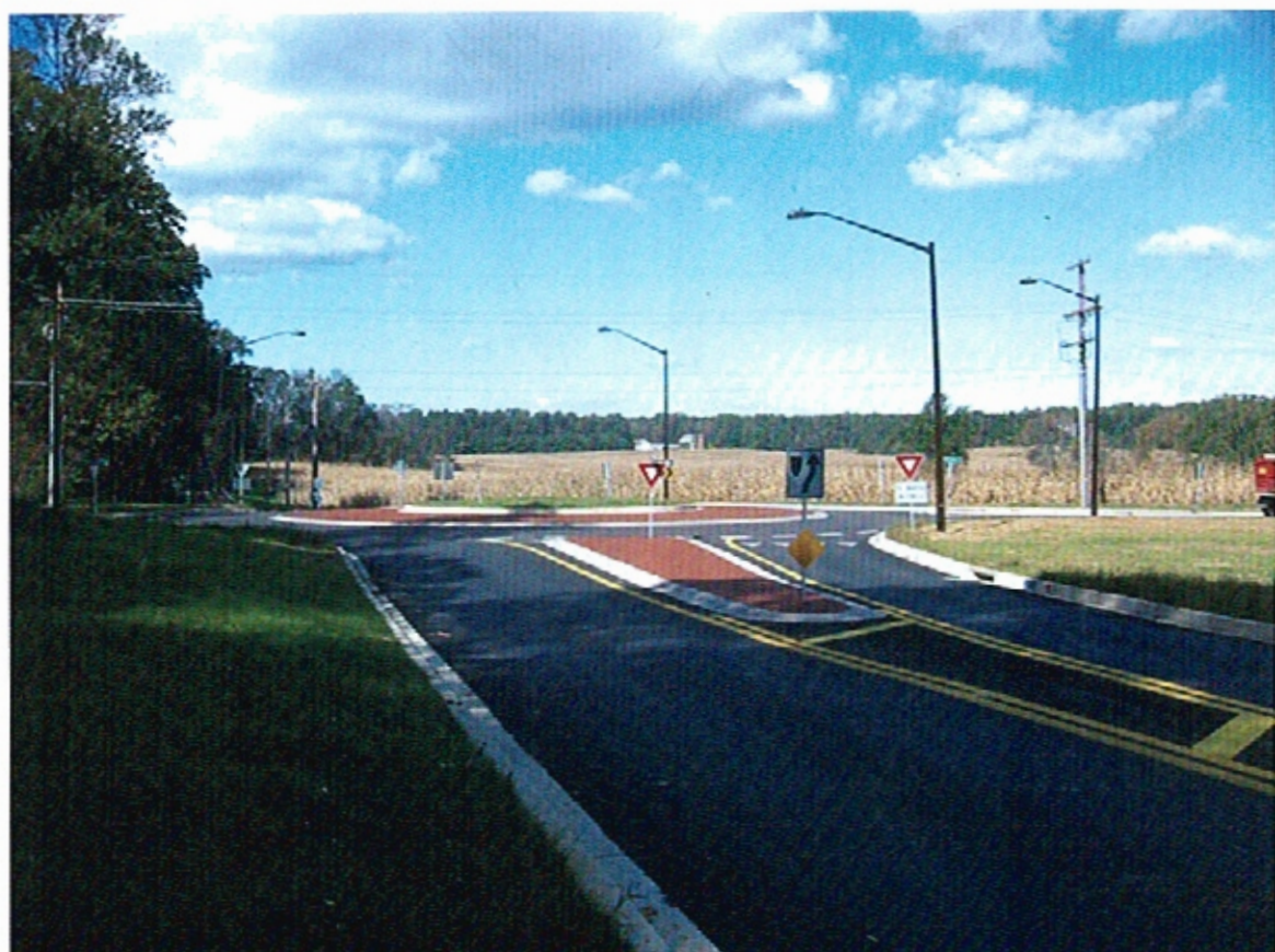
Shepard Roundabout, showing approach and lighting.
