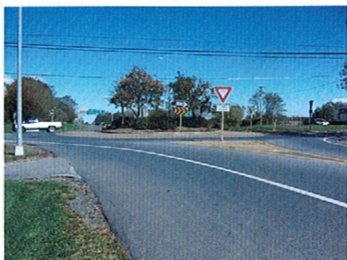
Lisbon Roundabout, south view
