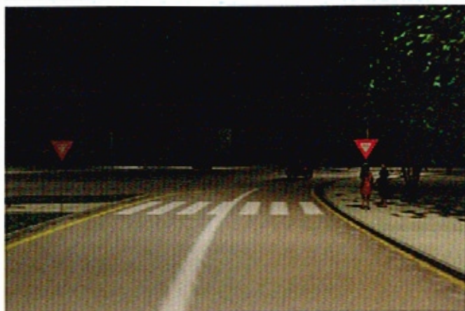
Lighting produced by a perimeter mounted lighting system with 8-250w hps luminaires shown at right, top and bottom.
