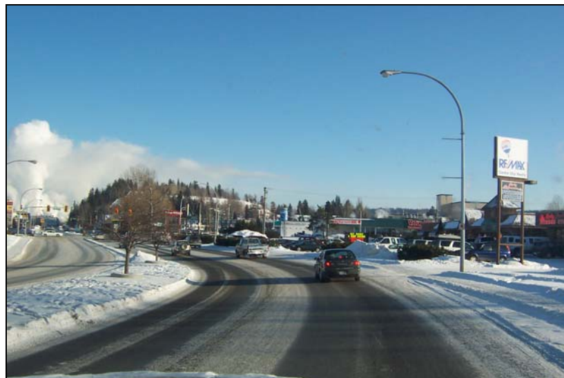
Figure 10 – 15 th Street Approaching Spruce Eastbound
